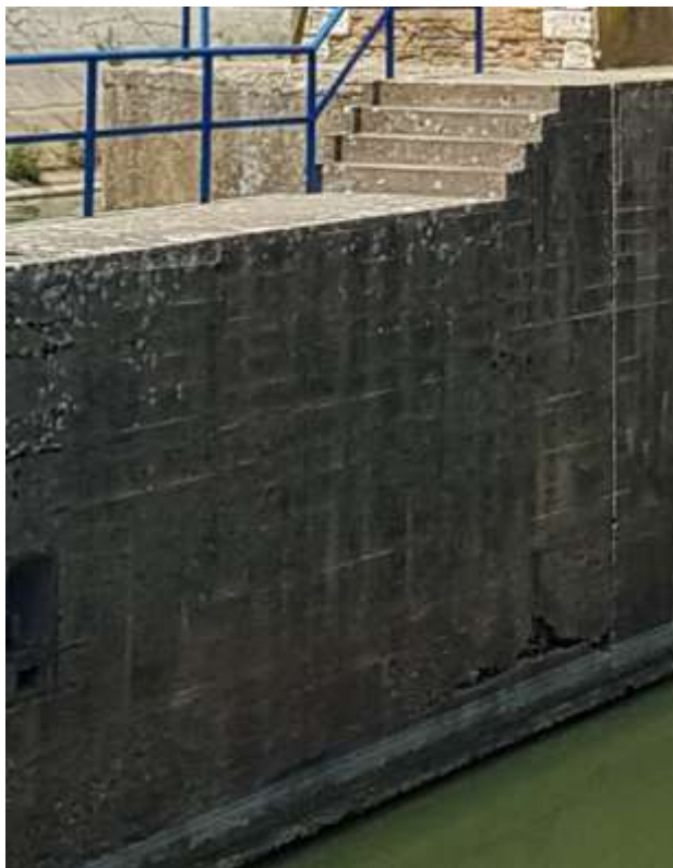
Damaged wall of the lower chamber of the ship lock
