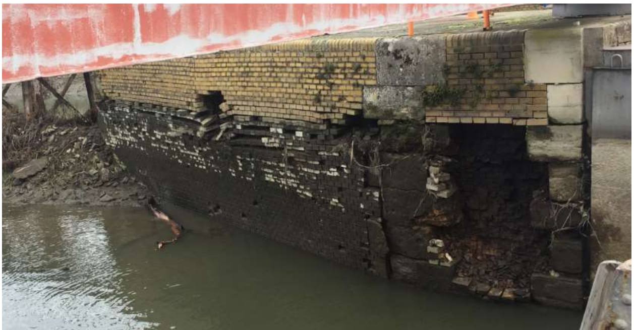
Damaged wall from the pier to the floodgate at a lower water level - close-up (December 2017)
