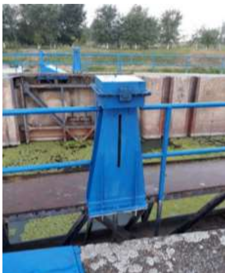
Figure 13. Manually driven flashboards of the lower door lifting/lowering mechanism
