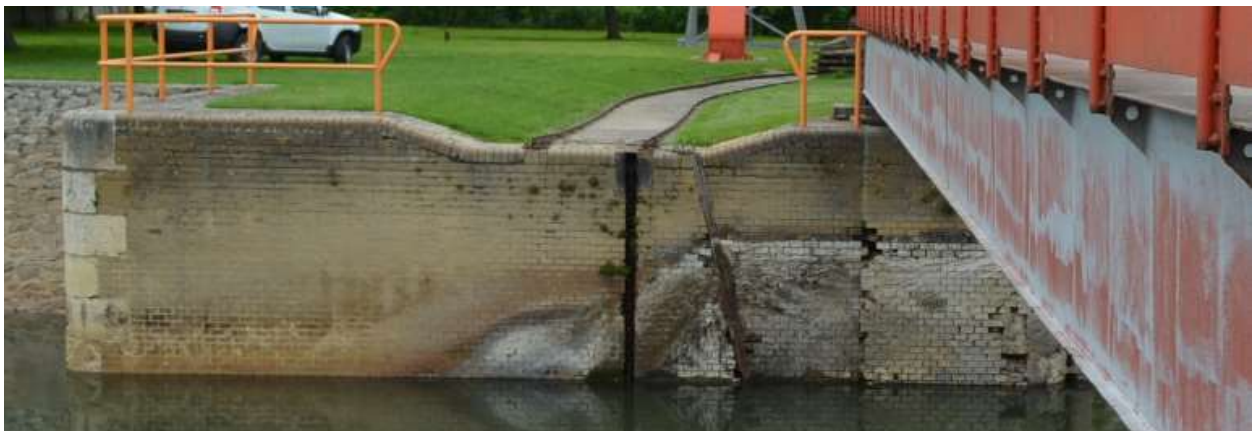
Damaged bank wall at the right bridge support (December 2017)
