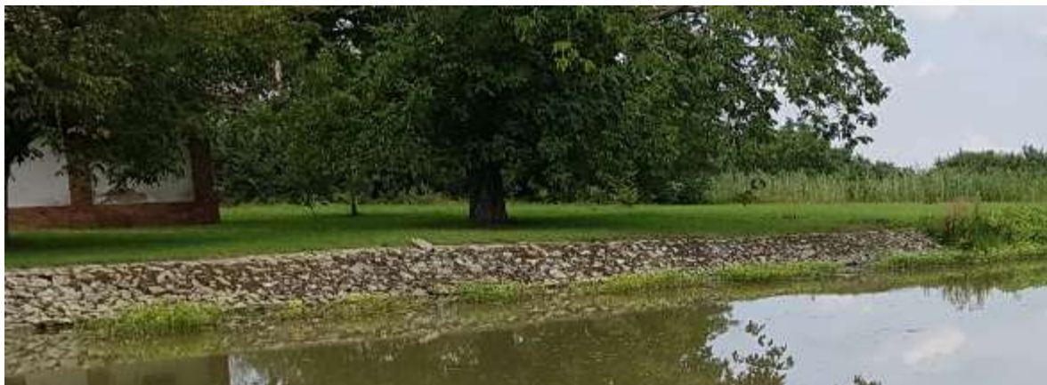
Damaged bank revetment
