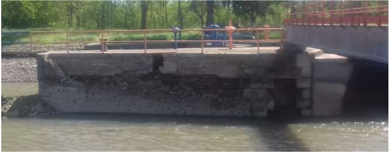
Damaged wall from the pier to the floodgate at a lower water level (April 2018)
