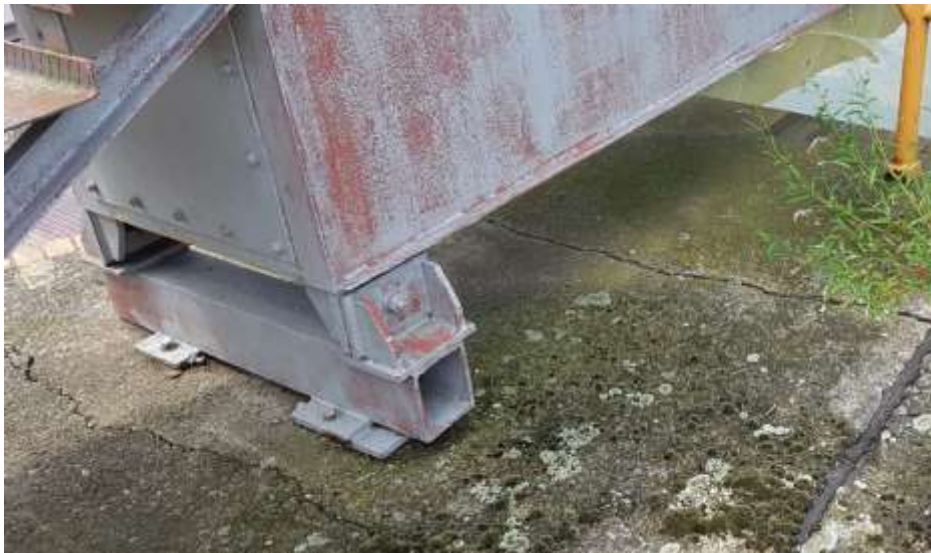
Subsidence of the left support of the pedestrian bridge on the ship lock wall - upstream view
