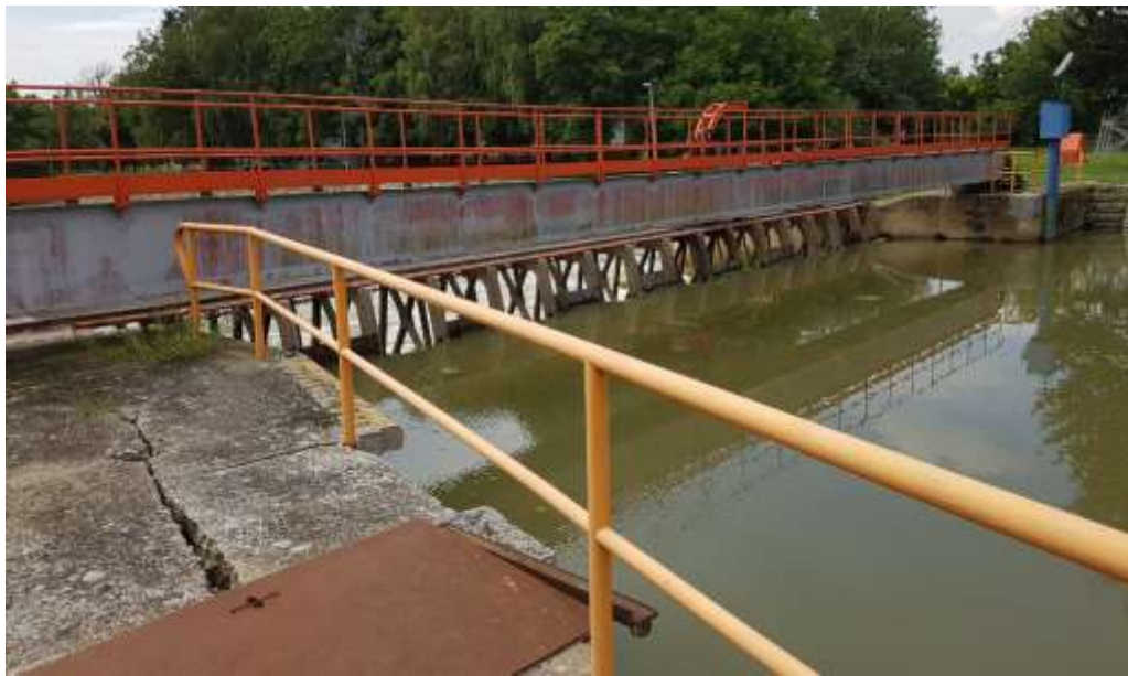
Damaged pathway on the right wall of the ship lock, in the area of the damaged wall from the pier to the floodgate
