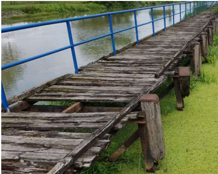
Damaged pier - close-up (August 2018)
