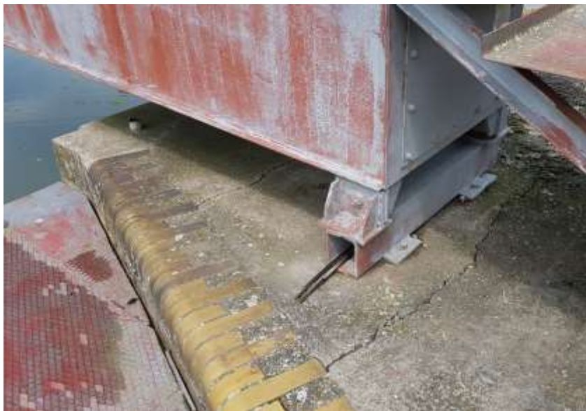
Subsidence of the left support of the pedestrian bridge on the ship lock wall - downstream view
