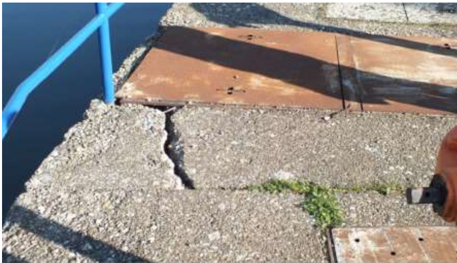
Damaged pathway on the wall of the ship lock
