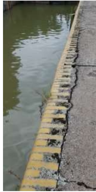
Damaged pathway on the right wall of the ship lock
