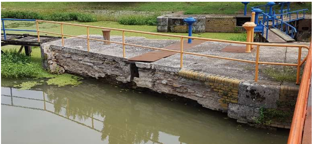
Damaged wall from the pier to the floodgate (August 2018)
