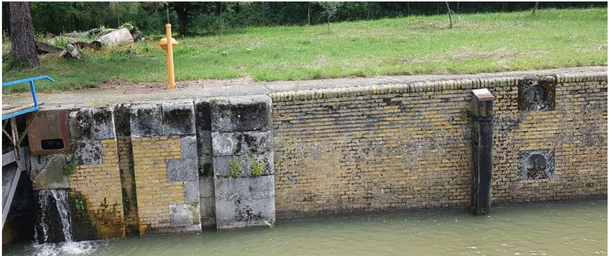
Damaged left wall of the ship lock chamber
