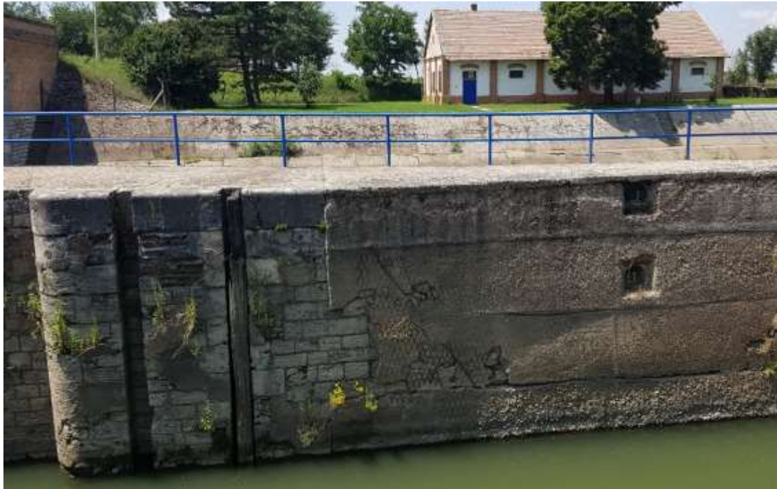
Damaged wall of the upper chamber of the ship lock
