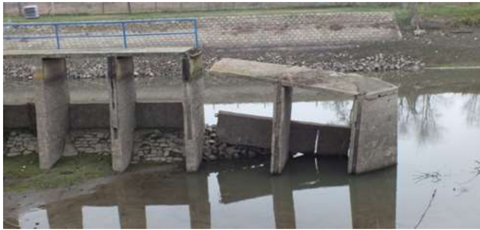
Damaged last two spans of the pier
