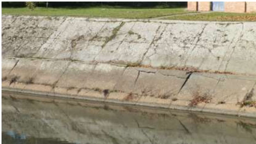
Damaged concrete lining of the canal
