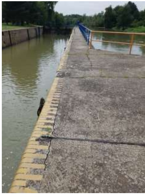
Damaged pathway on the right wall of the ship lock
