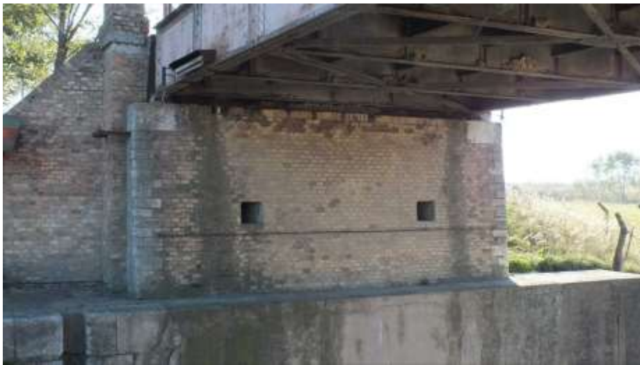
Damaged abutment
